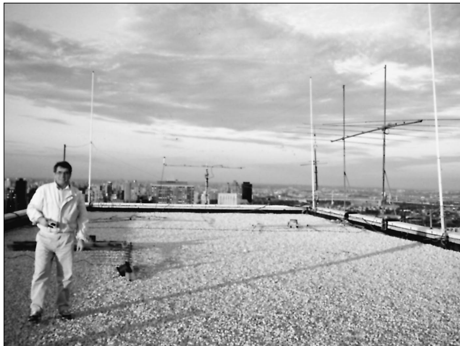
Dave Rosen, K2GM, chief operator at the 4U1UN/B beacon, on the roof of the United Nations building. The 14.1-MHz beacon antenna is a dipole at the far end of the roof.
